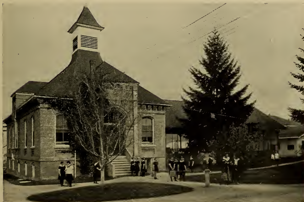
The Women's Gymnasium has been recently enlarged by the addition of a wing, which is so constructed as to provide all the advantages of exercise taken in the open air, combined with protection from rain.
